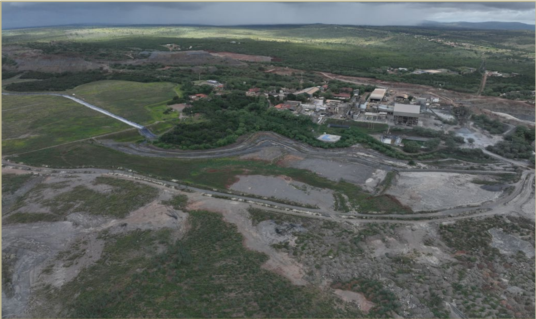
Figure 18-2: Site Photo of Facilities Layout and Infrastructure
