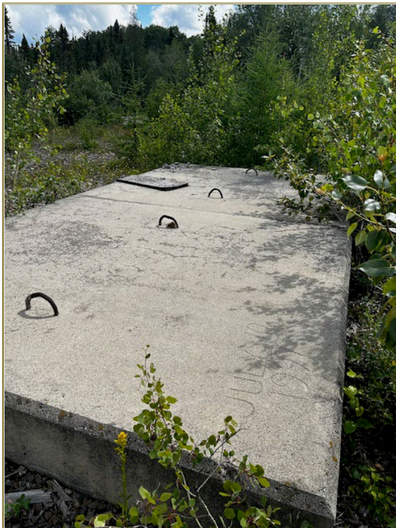
Figure 12-14: Mine Workings—Capped Jellicoe Shaft, Key Lake Property
