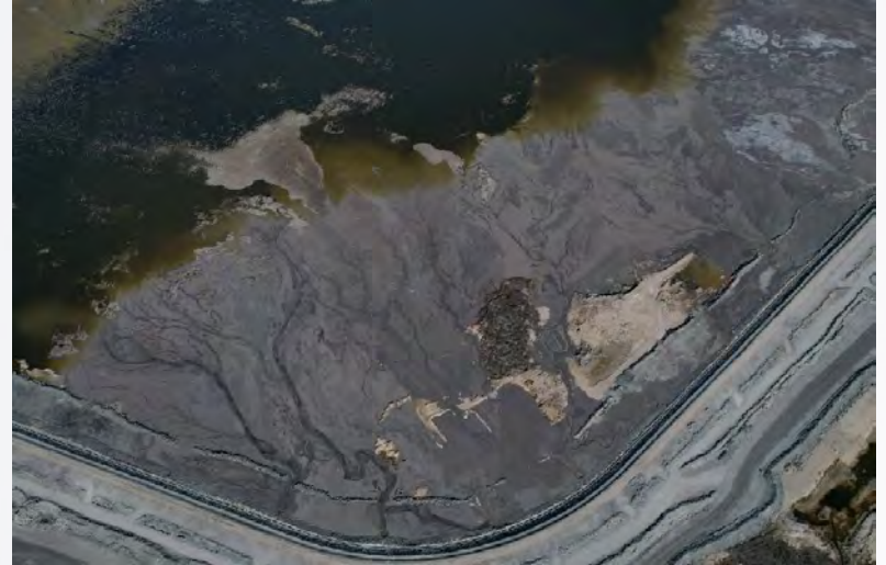
Overview of active tailings beach on Southeast Dam
