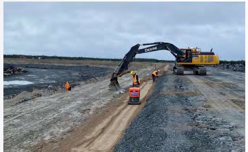
Construction of the till core and filters in 2024
