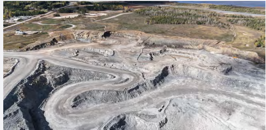
Legacy tailings excavated for disposal into TMF facility
