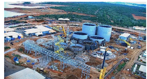
Leach tank installation
